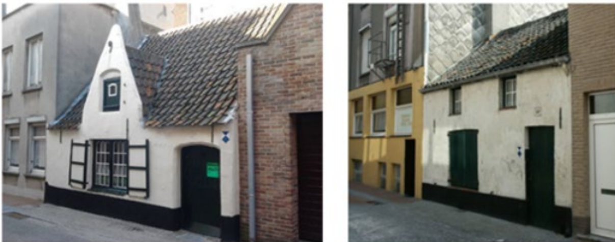
Figure 18: The Fishermen's Houses Majutte on the left and No. 27 on the right.
